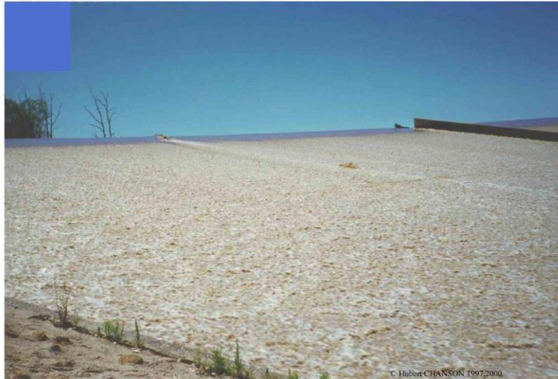
Turbulent air-water mixture on a chute
