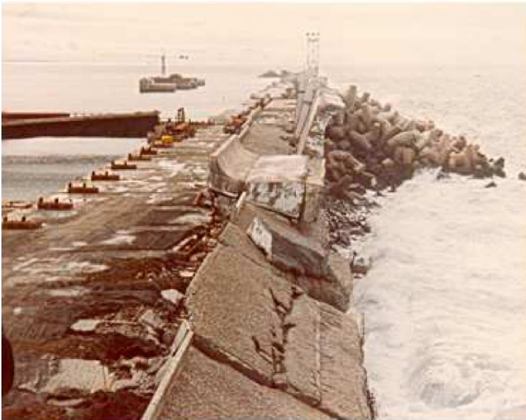
Images of destroyed Sines breakwater, 1978/9
