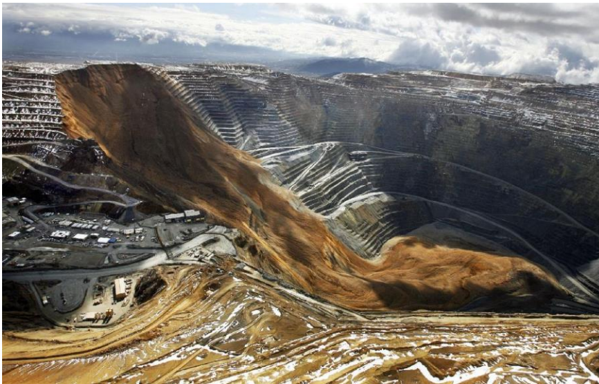
Bingham Canyon Mine landslide
